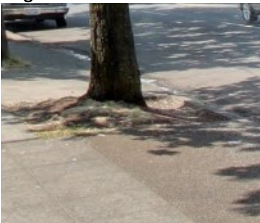
Example of tree pits with exposed roots
